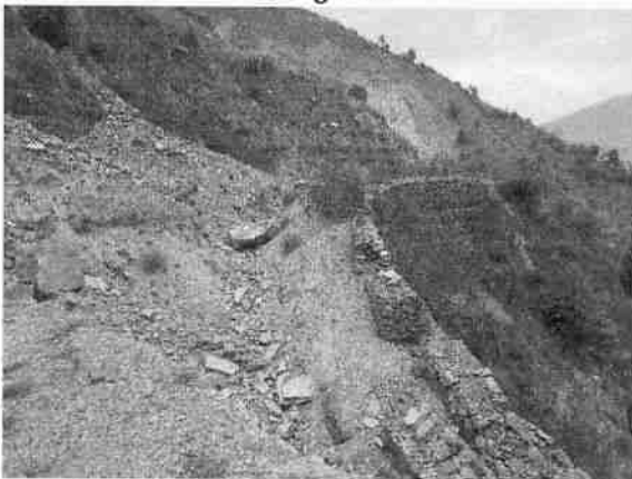
Road Block and Damaged Retaining Wall
