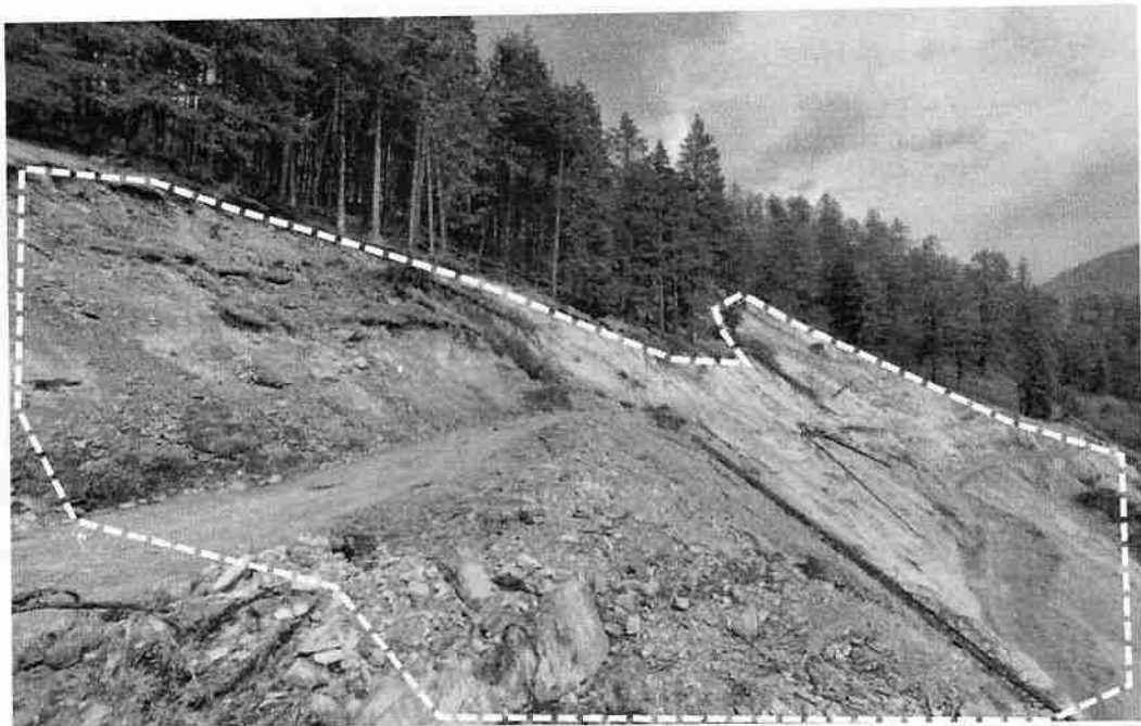
Figure 3: Slope failure (Circular failure) along the Sutol - Kanol road between KM 06 and KM 07.
