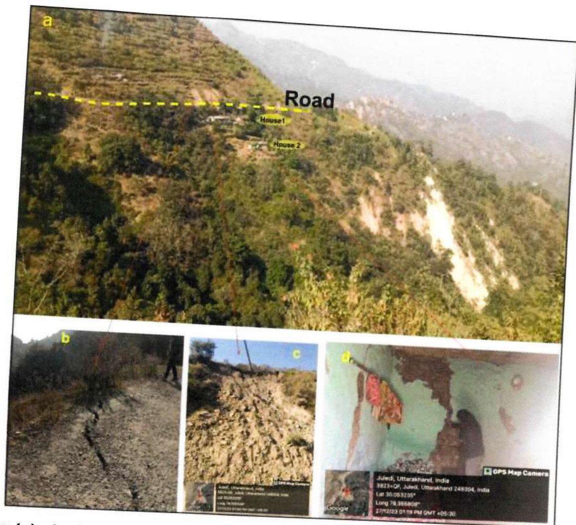
Figure 1 showing the position of landslide scarp in Spot 1 along with road cracks and poor construction of house-2 in which fallen plaster has seen
