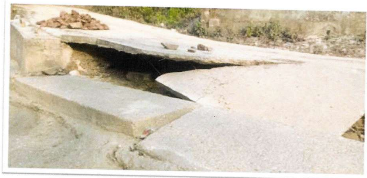
Figure 17 exhibiting the erosion and wrong constructional practices
