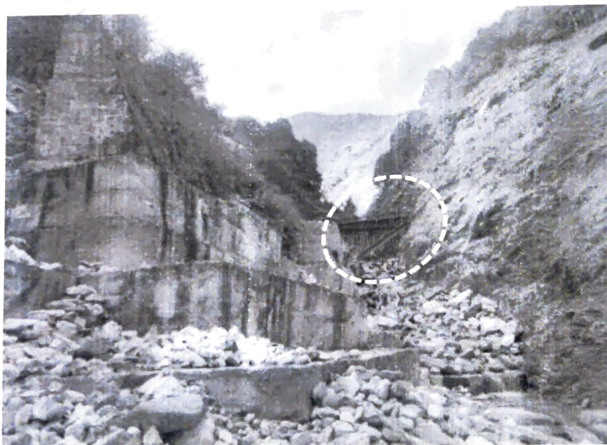
Figure 5: Figure shows the destruction of the bridge caused by the intense discharge during the monsoon.
