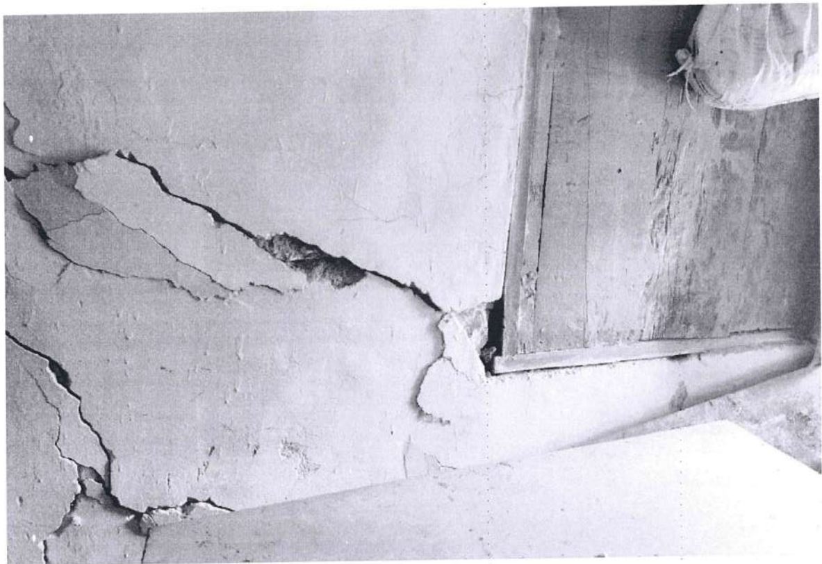
Figure 5: Cracks observed in building structures during field inspection, suggesting potential differential settlement or ground movement.
