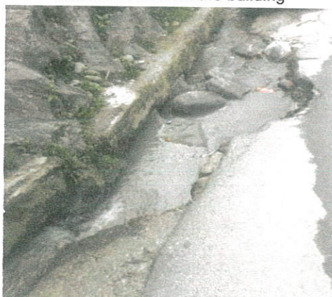
Broken drain at Main Bazar
