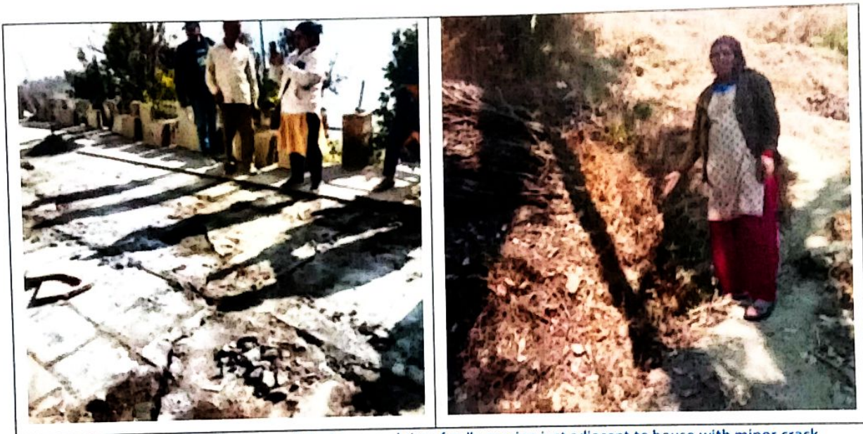
Figure 8 exhibiting broken tiles in one of the house and site of gully erosion just adjacent to house with minor crack (note that such cracks do not appear inside the house and only restricted in small portion of outside of house)
