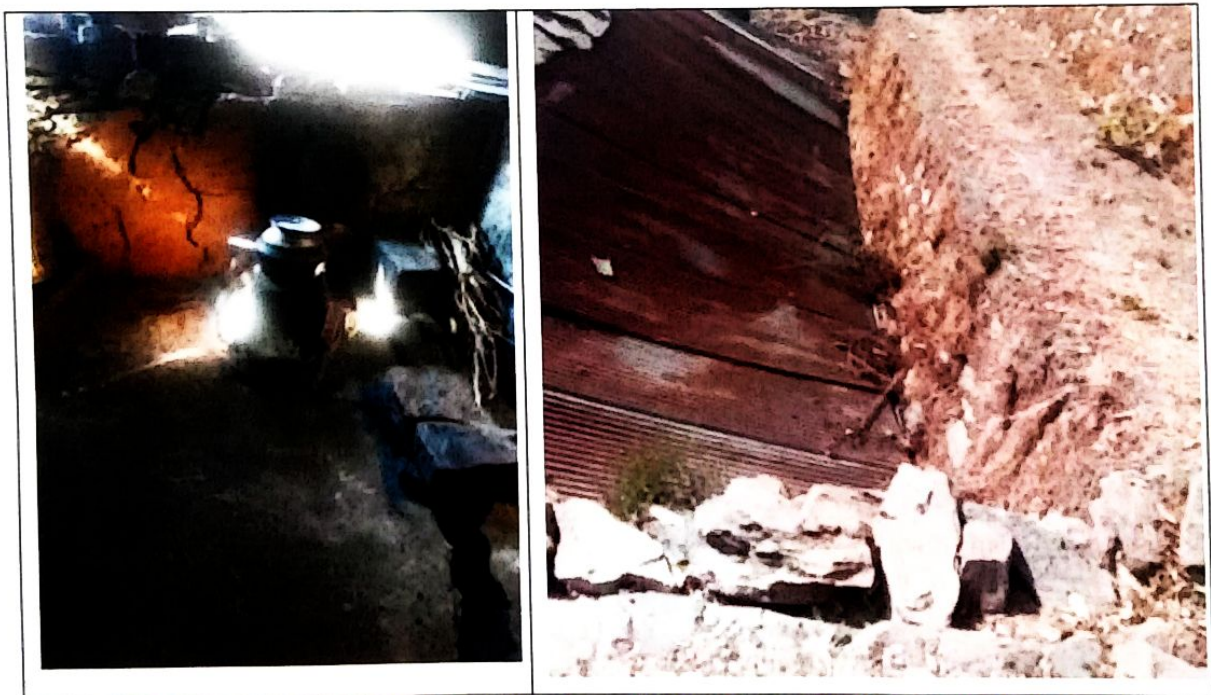
Figure 3 : (left) widen crack on ground of a house just above village metalled road located at N 30.640540° lat and E77.830775 longitude , (right) just above the crack, a tinshed is placed that ingress the rainwater inside the closed room without having proper drain out system
