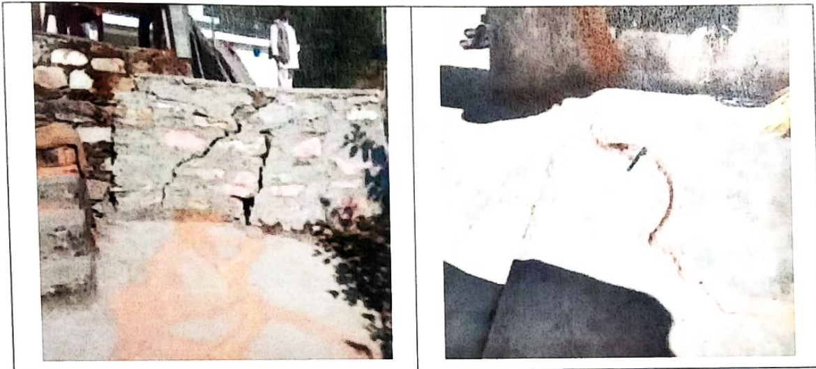
Figure 4 exhibiting unusual crack pattern on concrete base which is filled by mud and broken newly constructed retaining wall
