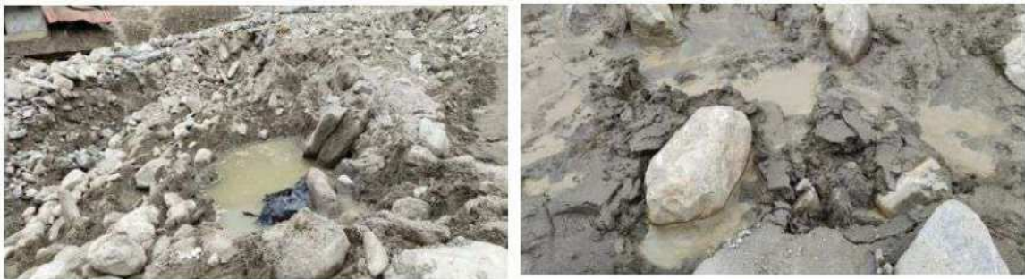
Fig. 13: The water getting filled-up during the manual excavation showing the presence of underground water
