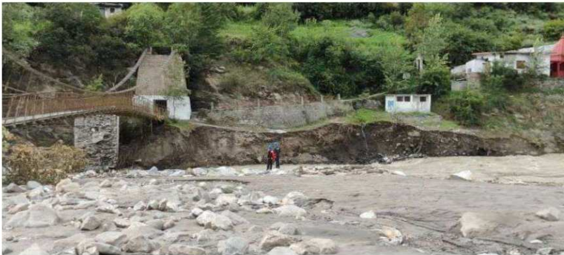
Fig. 14: Impact of water on the right bank of the river damaging the foot bridge connecting Dharali to Mukhba
