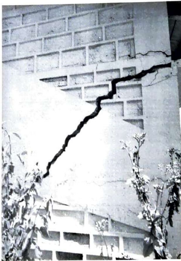
Figure 3: Cracks observed in building structures during field inspection, suggesting potential differential settlement or ground movement.
