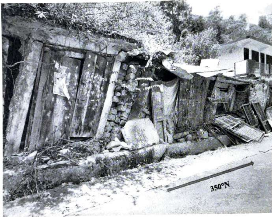
Figure 4: Structural cracks observed in buildings at Baldev Market, highlighting signs of damage possibly due to subsidence or geotechnical failure
