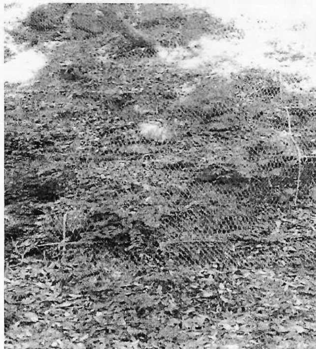
Figure 12 GI wire net in less vegetation area
