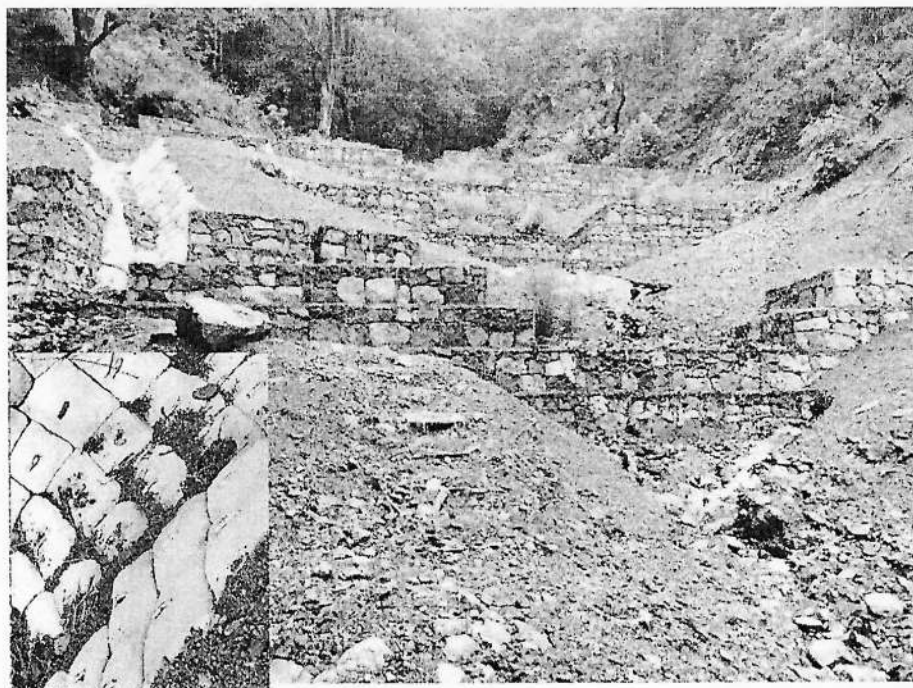
Figure14. gabion networking with Geo bag channel filled with local soil.
