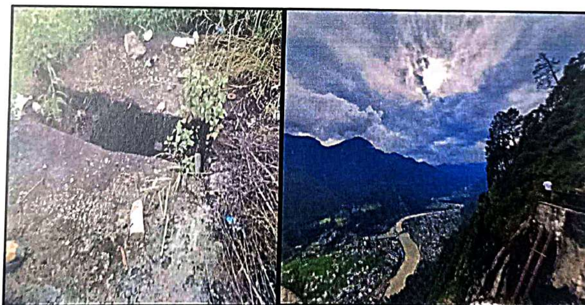
Figure 11: The catch drain is choked require to be opened at platform at EL \pm 1660m.
