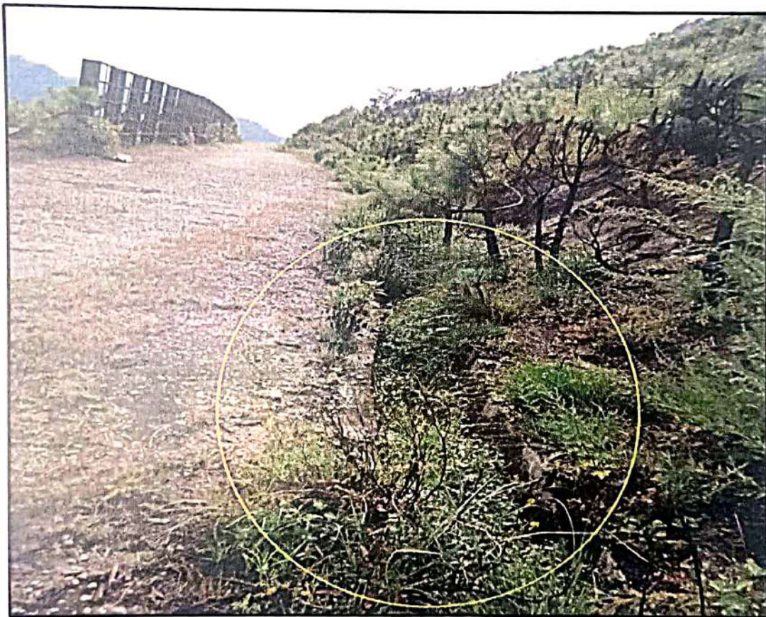
Figure 9: Choked catch drain
