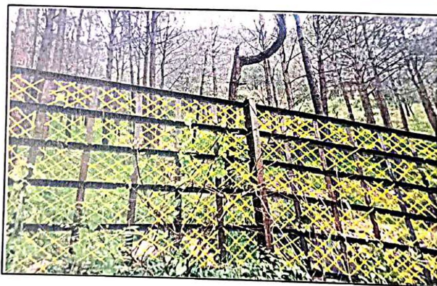
Figure 14: Design of chain link fabric to be welded behind the existing barricade.
