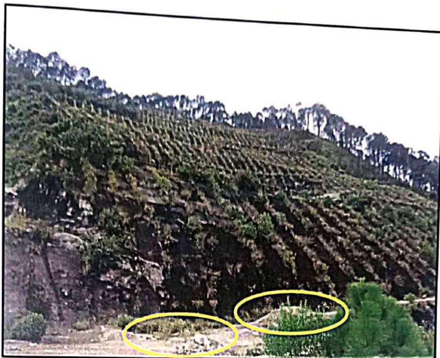
Figure 12: Construction materials sand and boulders were left at the edge of the bench. It has to be removed
